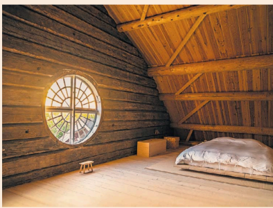
The spruce-timber roof is a replica of the 18th-century barrel roof, with 12-metre-long beams cut from single trees
